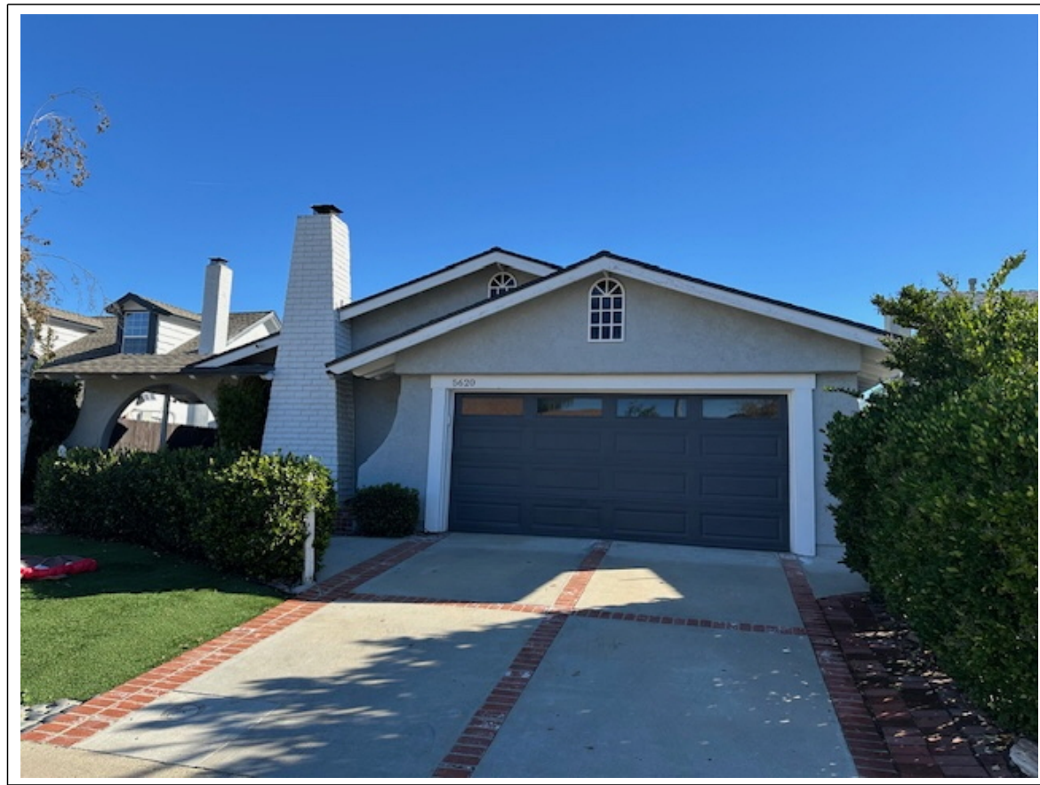
FRONT DRIVEWAY VIEW 2026-01-30 ②
