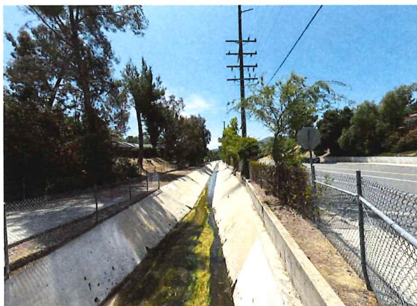
Figure 3: Liberty Canyon - Existing Condition
