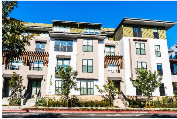
FIGURE 28(A). URBAN RESIDENTIAL – ELEVATOR
