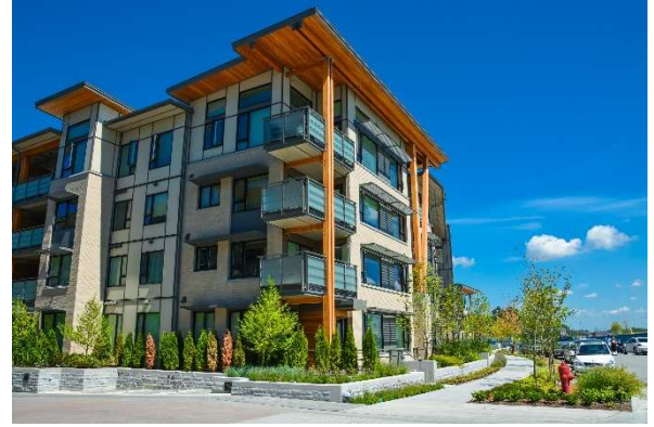
FIGURE 28(B). URBAN RESIDENTIAL - ELEVATOR
