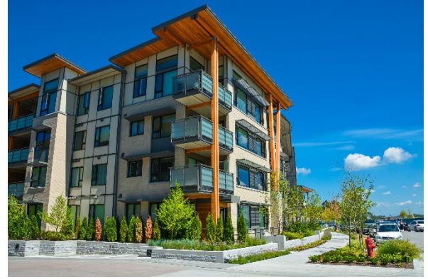
FIGURE 28(B). URBAN RESIDENTIAL - ELEVATOR
