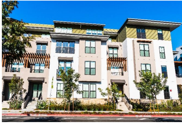
FIGURE 28(A). URBAN RESIDENTIAL – ELEVATOR
