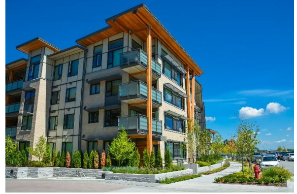
FIGURE 28(B). URBAN RESIDENTIAL - ELEVATOR
