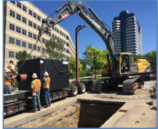
Figure 5: Butterfly Valve Vault Install
