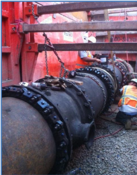
Figure 6: Large Diameter Water Repairs
