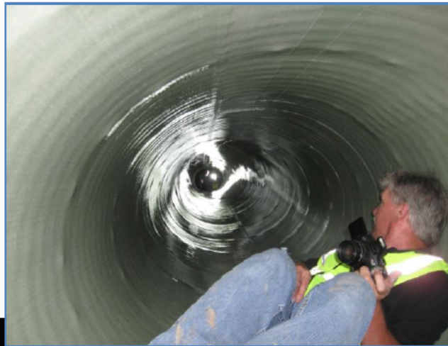
Figure 20: UV CIPP Lining of CMP Storm
