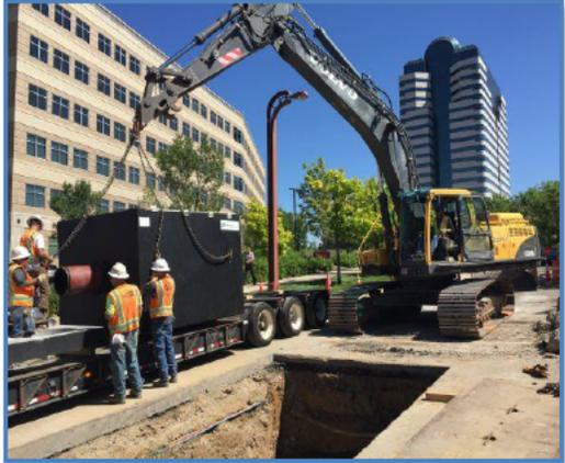
Figure 5: Butterfly Valve Vault Install
