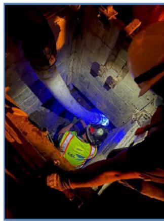
Figure 26: LED Lateral Lining
