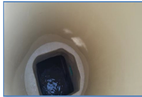
Figure 24: Manhole Rehabilitation
