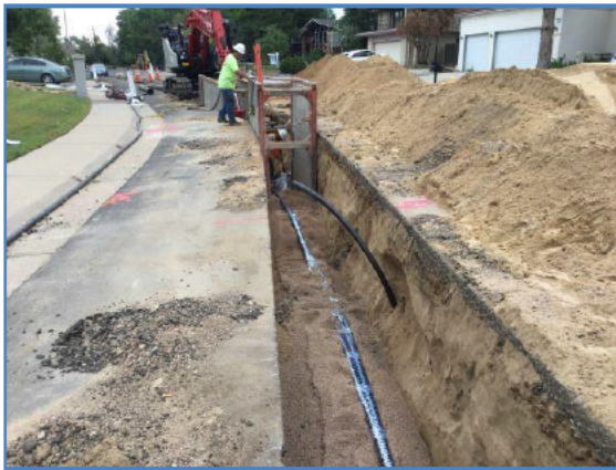
Figure 2: Open Cut Water Line R & R.
