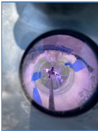
Figure 25: UV Cured MH Rehab
