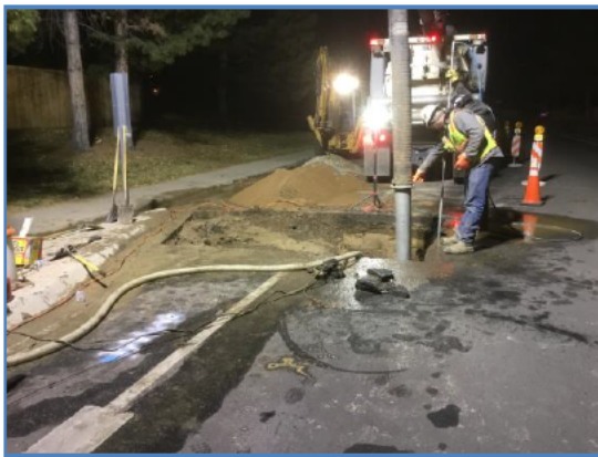
Figure 30: Emergency Response Water Break
