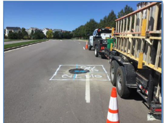
Figure 29: Water Break Layout and Crew Setup
