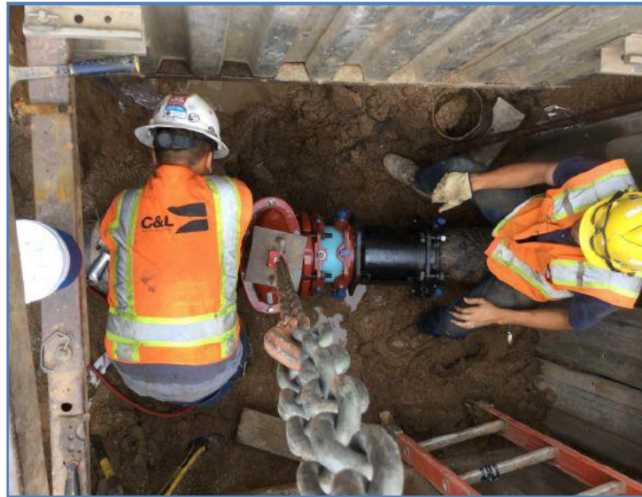
Figure 7: Valve Repairs/Replacements
