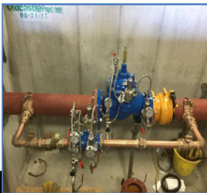
Figure 8: PRV Installation
