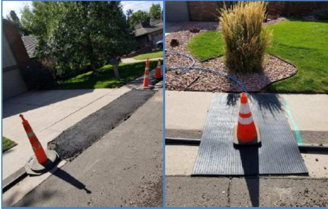
Figure 4: Temporary Water Example
