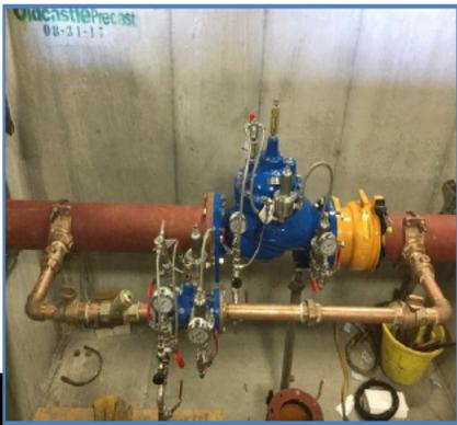
Figure 8: PRV Installation
