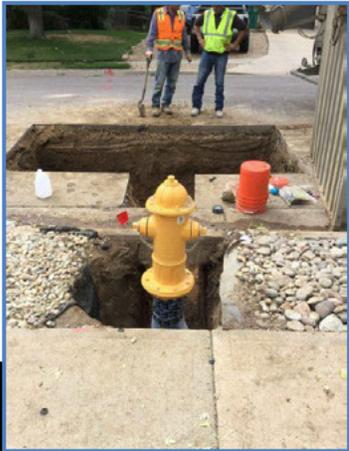
Figure 9: Fire Hydrant Replacement
