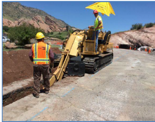
Figure 3: Water Line Install with Trencher
