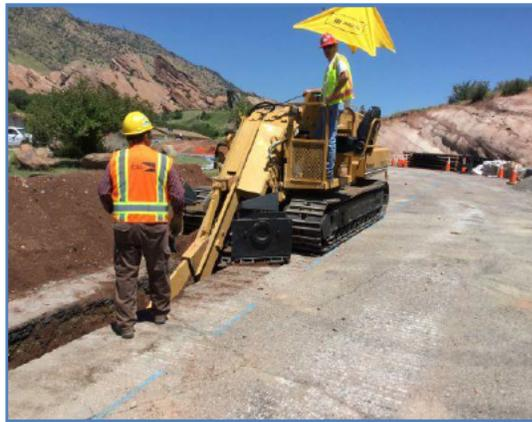
Figure 2: Open Cut Water Line R & R.
