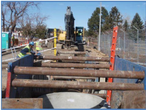
Figure 17 + 18: Storm Sewer - New Installations
