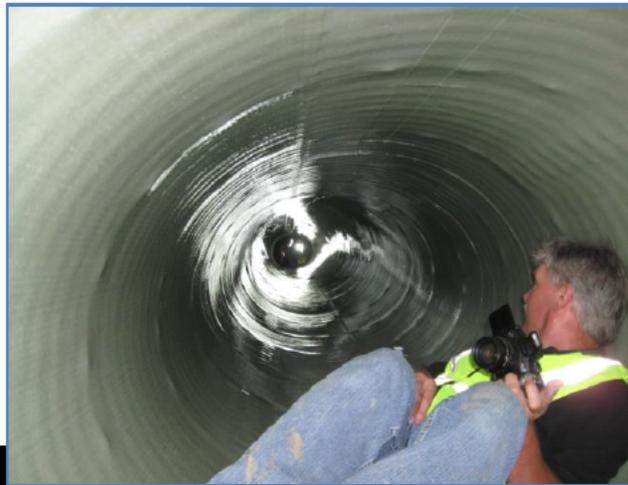
Figure 20: UV CIPP Lining of CMP Storm
