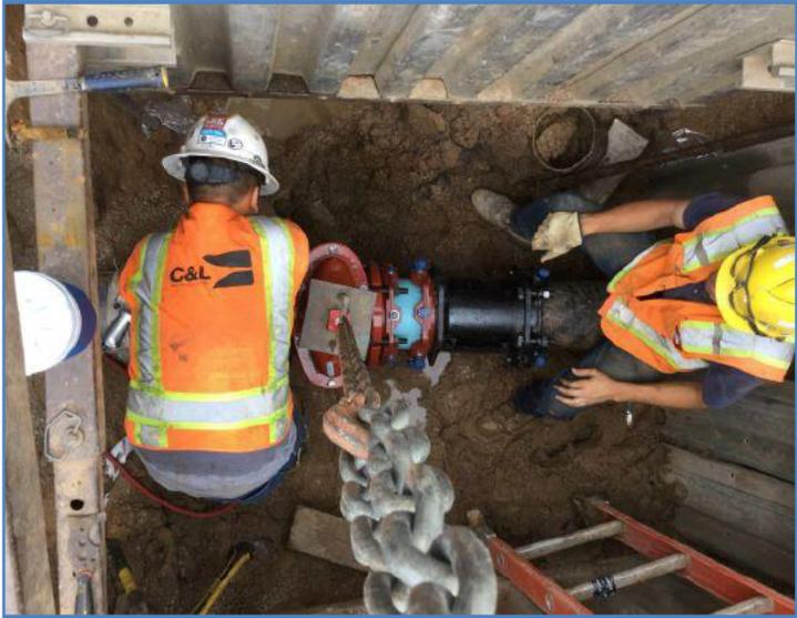
Figure 7: Valve Repairs/Replacements
