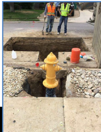
Figure 9: Fire Hydrant Replacement
