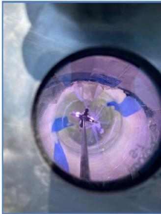
Figure 25: UV Cured MH Rehab
