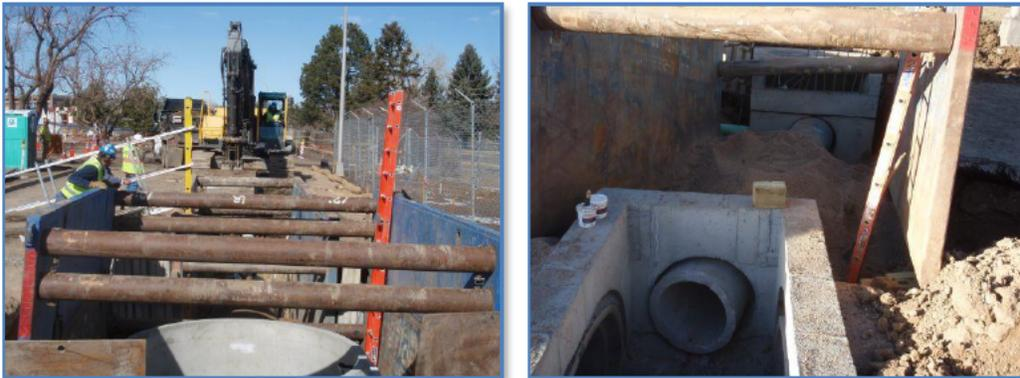
Figure 17 + 18: Storm Sewer - New Installations
