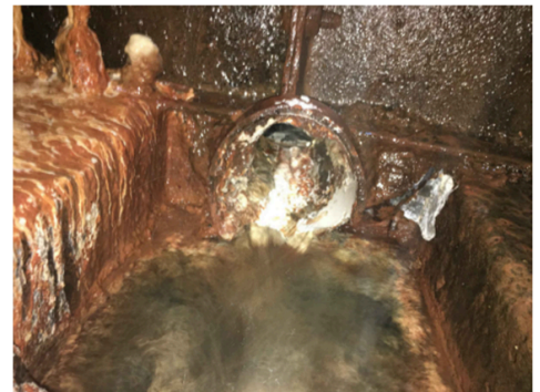
SOUTH TOE DRAIN AFTER CLEANOUT
