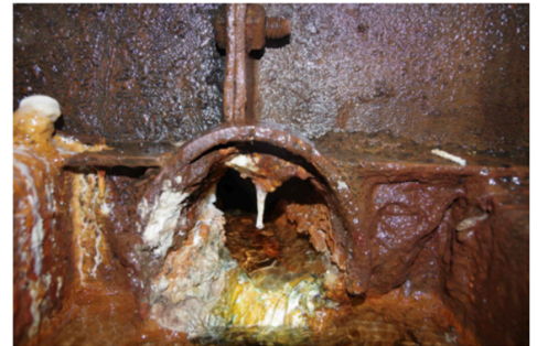
SOUTH TOE DRAIN BEFORE CLEANOUT
