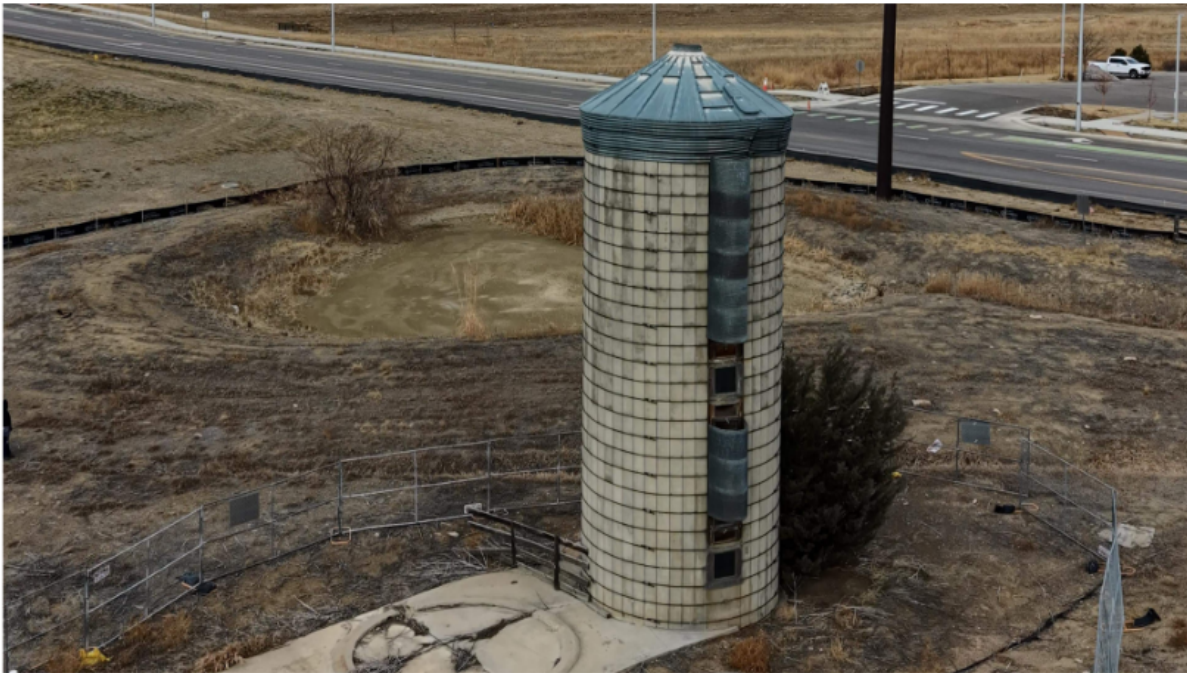
Nordstrom Silo, southeast elevation
