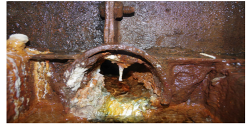
SOUTH TOE DRAIN BEFORE CLEANOUT
