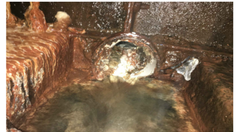
SOUTH TOE DRAIN AFTER CLEANOUT
