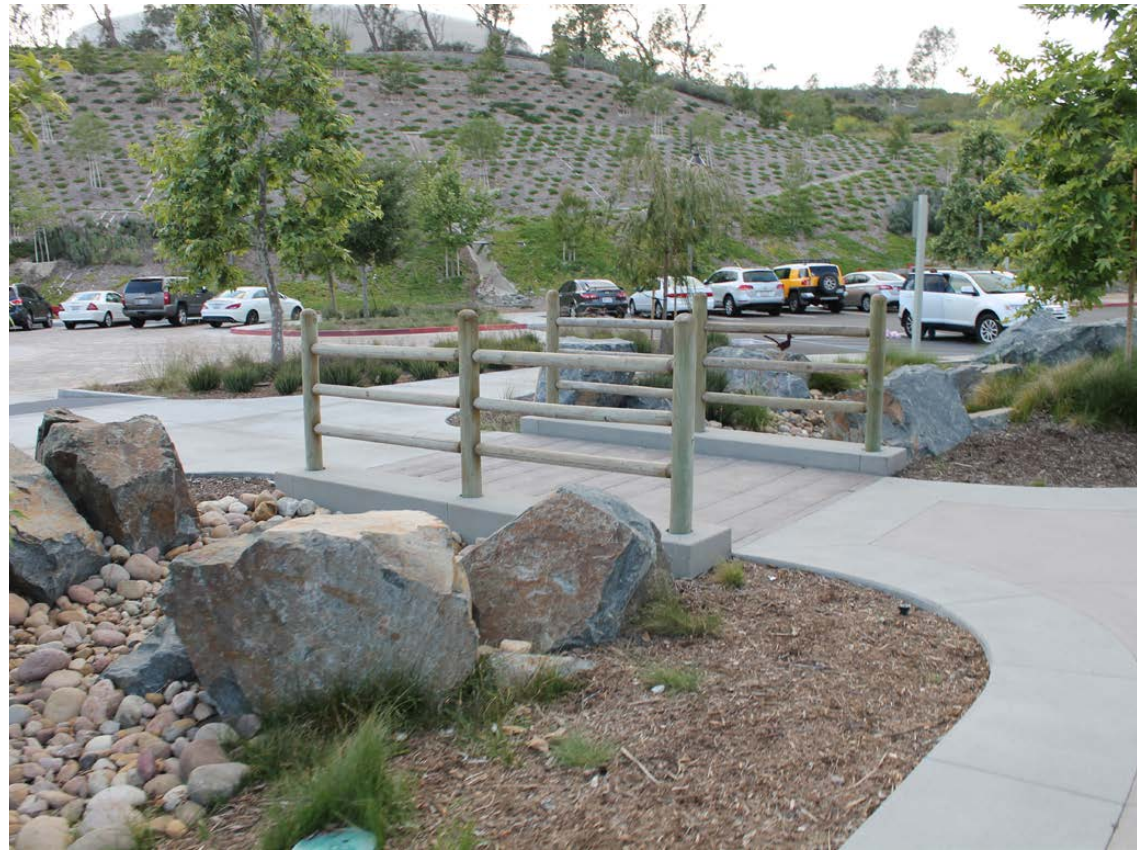
Bioswale and Bridge
