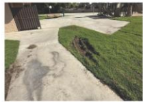
A. LACK OF MAINTENANCE TRUCK ACCESS
