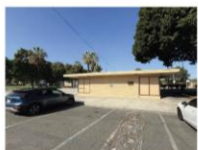
3. EXISTING COMMUNITY BUILDING WITH PUMP HOUSE
