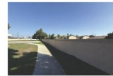
7. LOW PERIMETER WALLS
