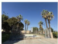
C. EXISTING WADING POOL (NON-OPERATIONAL)
