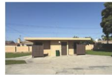
5. EXISTING RESTROOM FACILITY
