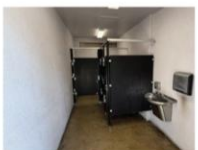
6. EXISTING RESTROOM FACILITY
