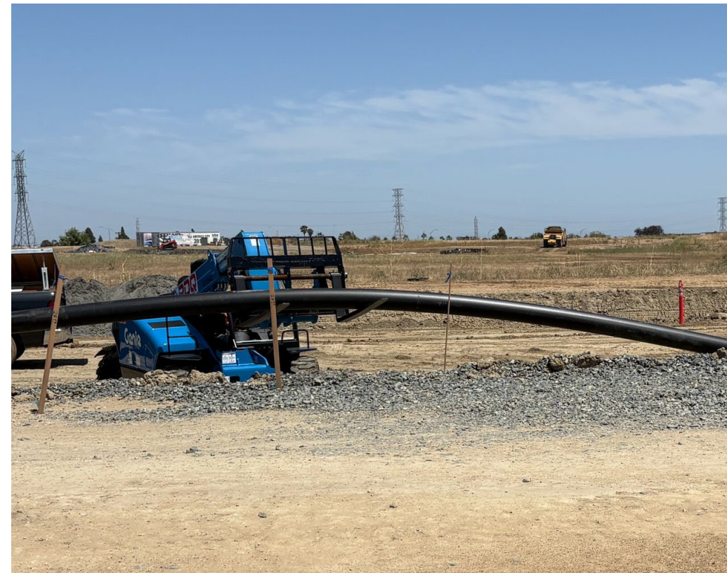
GCCS Header Line Installation - View North at Lenardo & Stamps
