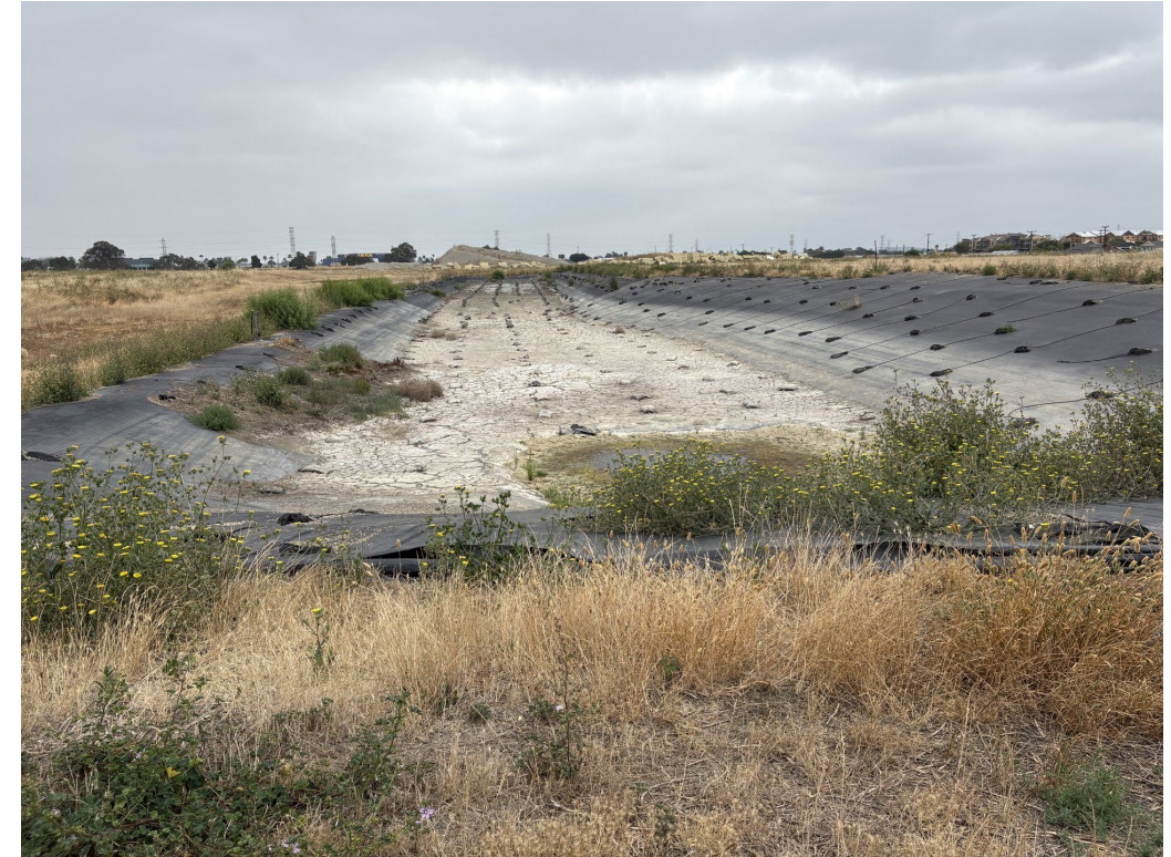
Basin C: View North
