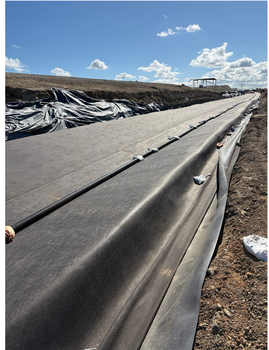
Cell 1 Buffer Zone Stormwater Liner. View East on Lenardo from Main Street
