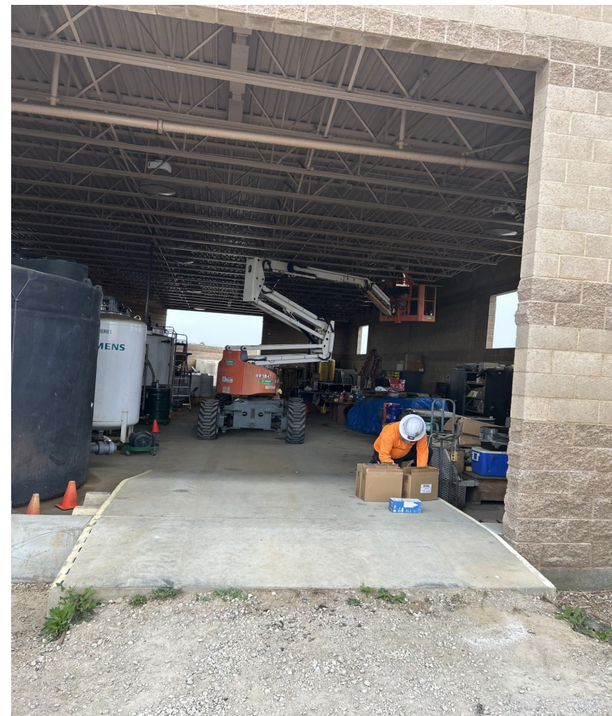
Manlift/Personnel Replacing Lights in LOC
