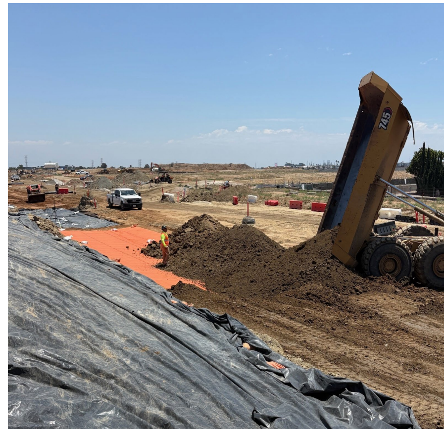
Placing Backfill On Top of Cell 1 Buffer Zone. View East on Lenardo Drive
