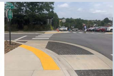
Short-term, low-cost pilot projects like painted curb extensions and crossings have led to permanent intersection improvements in Fayetteville since the inception of this program in 2016.
