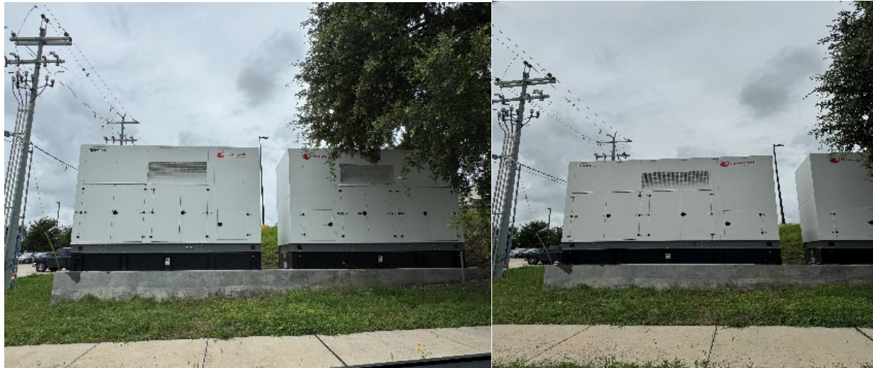
(Pictures above were taken on June 2, 2026)
