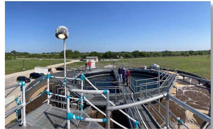
CCMA South Plant 0.5 MGD, Phase I
