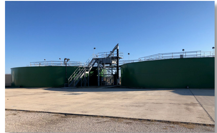
CCMA South Plant 0.5 MGD, Phase I
