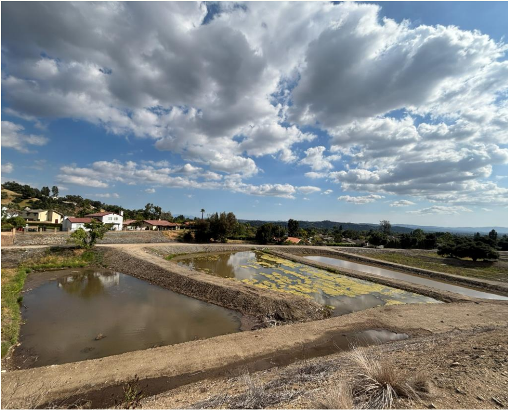
Dalton Wash Spreading
