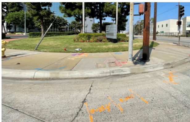
Constructability Review showing DigAlert markings and GTS marking of proposed foundations
