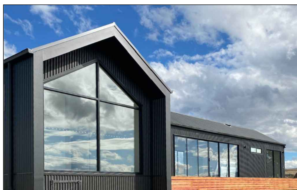
MODERN/CONTEMPORARY GABLE ROOF RUNS HOME.
