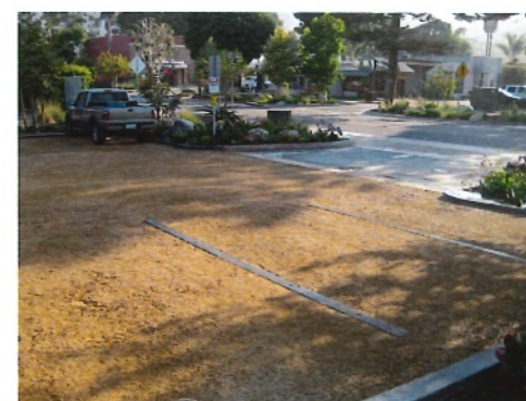
Example of pervious paving for parking areas
