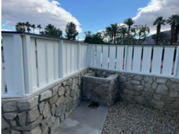
West perimeter wall, looking southeast, shows original rock detail and burn pit
