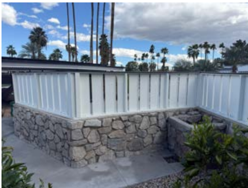
West elevation, looking southeast. Exterior perimeter wall shows angles
