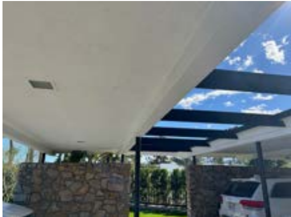
Porte cochere, looking south, shows opening in walls and the 'positive-negative' space of walkway, plus 'floating' roof above walls
