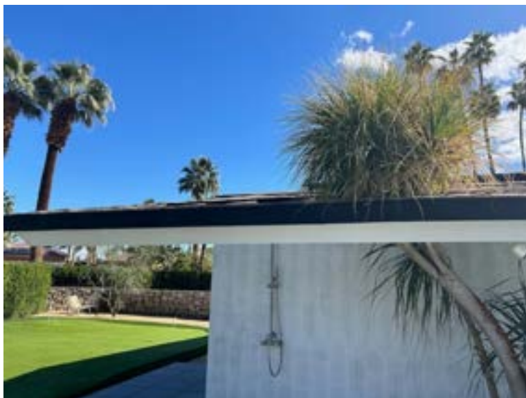
Northeast corner wall and roof opening
