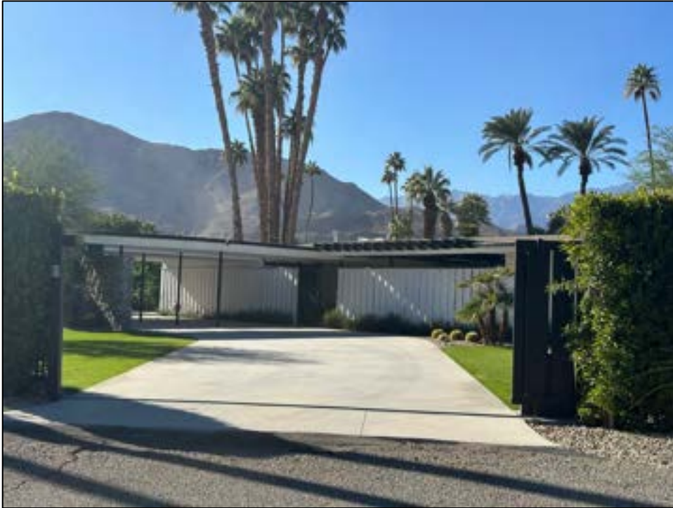
View of southeast (front) elevation. (71-076 Country Club Drive_3)
