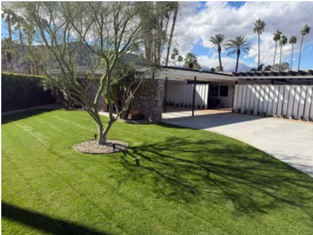
Porte cochere outer rock wall elevation: image shows both sections of wall with vertical opening between both walls. Image February 2026.
