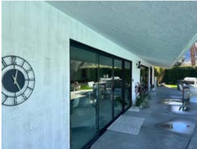
North elevation shows walls of windows and roof overhang
