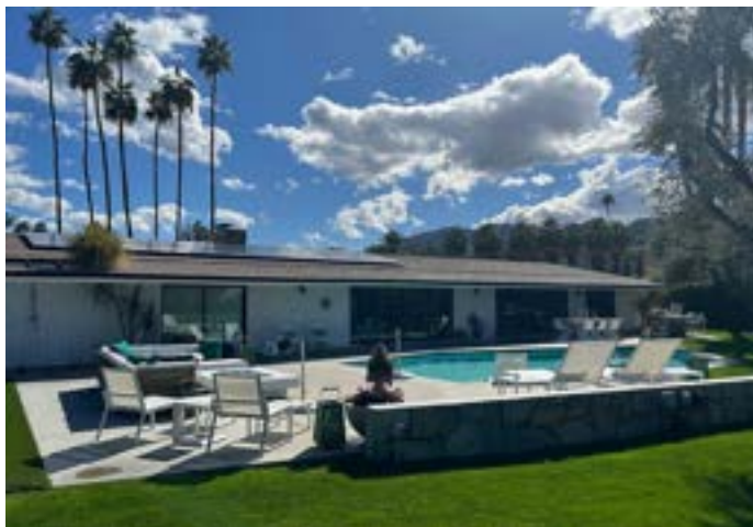
Rear, north elevation, looking southwest
