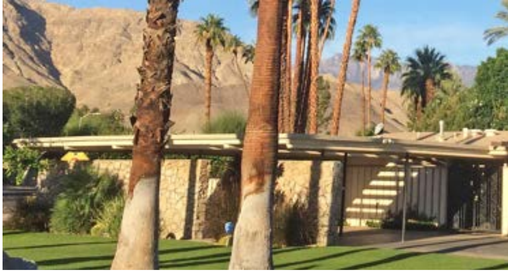
photo from 2018, wall is unchanged today
