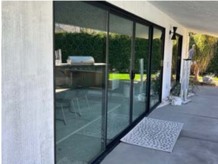
Northwest corner, overhang, windows, stucco detail
