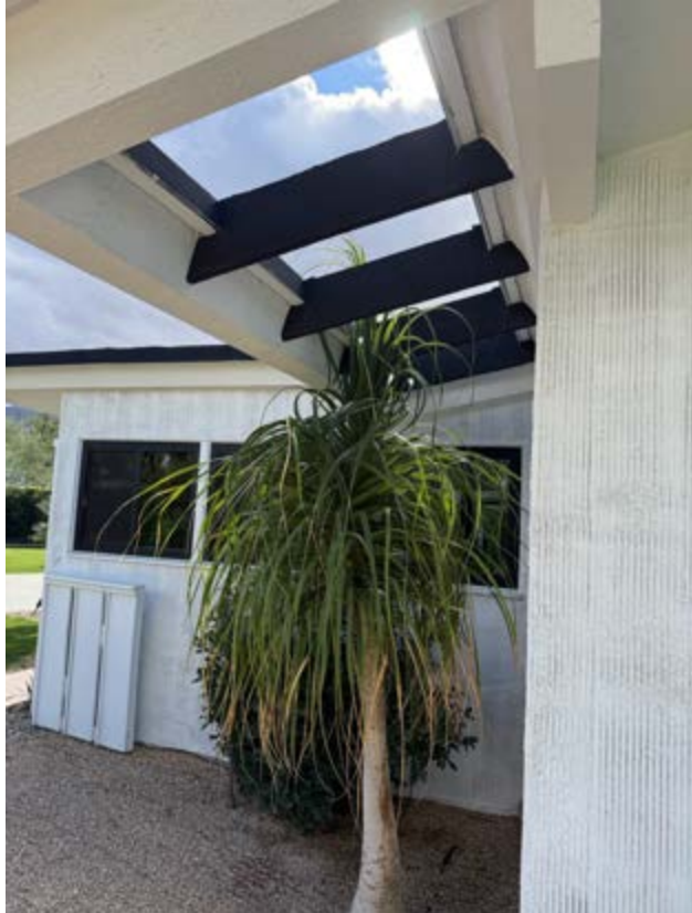
Roof opening, southeast corner
