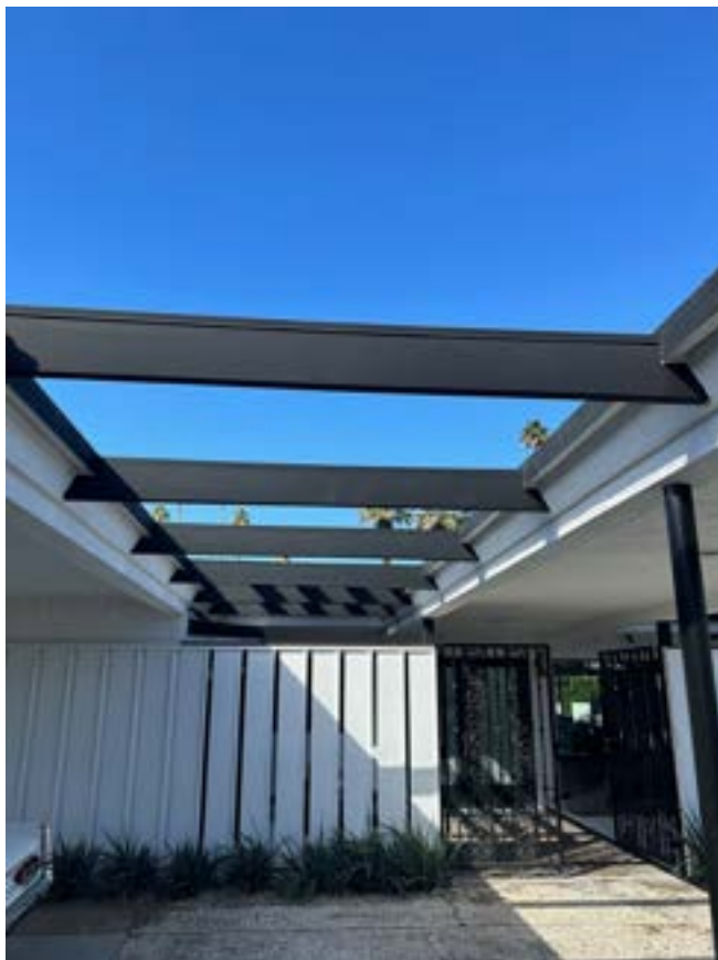
Lattice-beam open-air walkway adjacent to covered walkway leading to entrance
