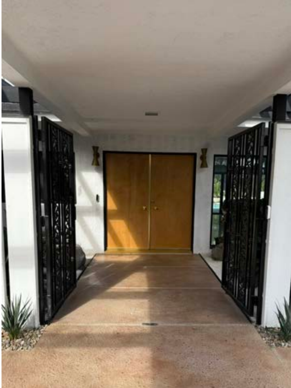
Entry pathway detail and custom birch front doors with 5" backsets.
