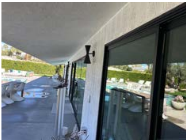
North elevation, windows, overhang
