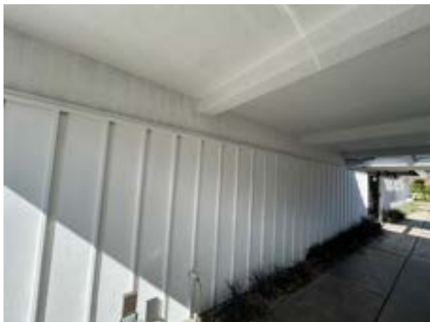
Southwest corner shows board & batten vertical louver continuation under porte cochere
