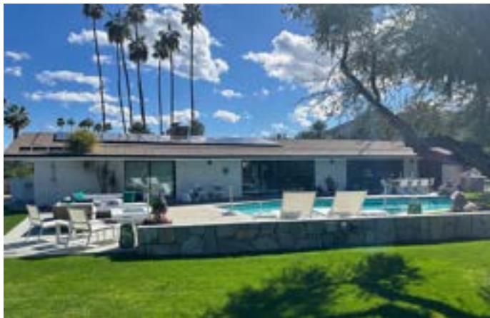
Rear, north elevation, pool, terrace wall
