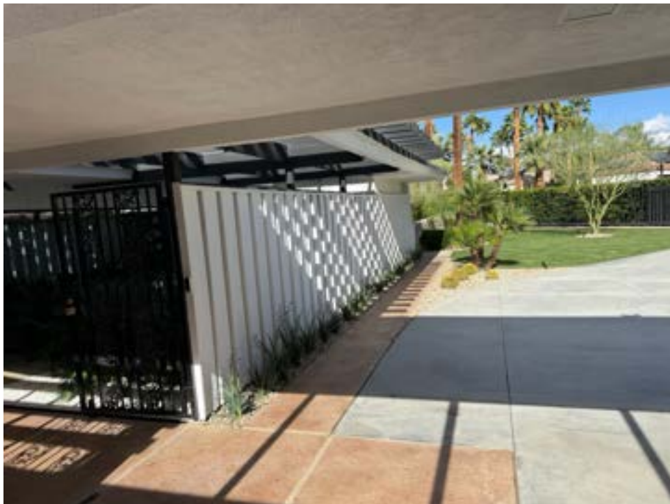
Row of vertical louvers to right of entry, that screen entry lanai, and pathway looking east
