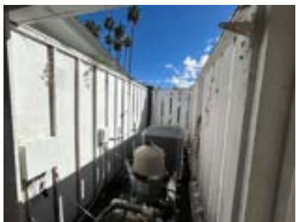
West elevation equipment area with board & batten, vertical louvers
