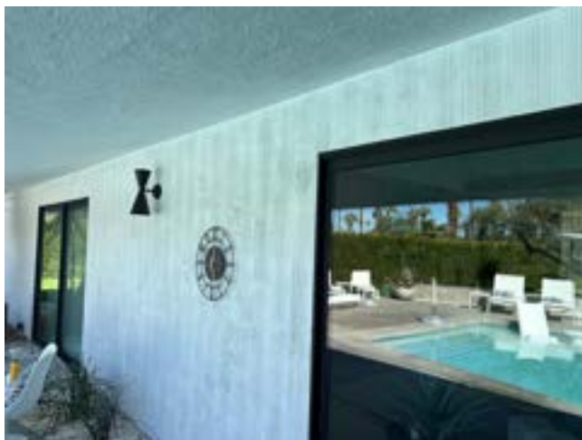
North elevation overhang, windows, stucco details
