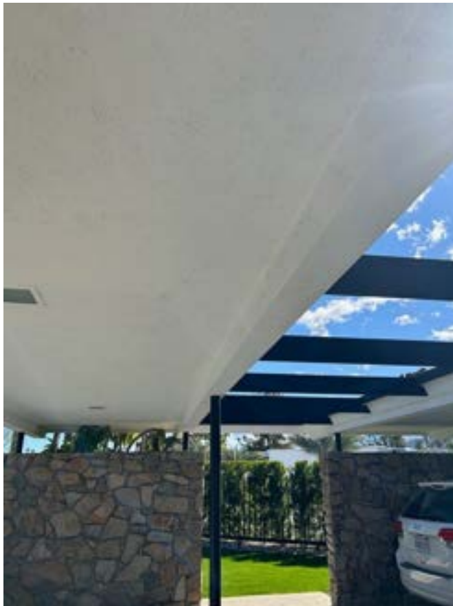
Porte cochere, looking south; covered and open walkway; opening between two rock walls
