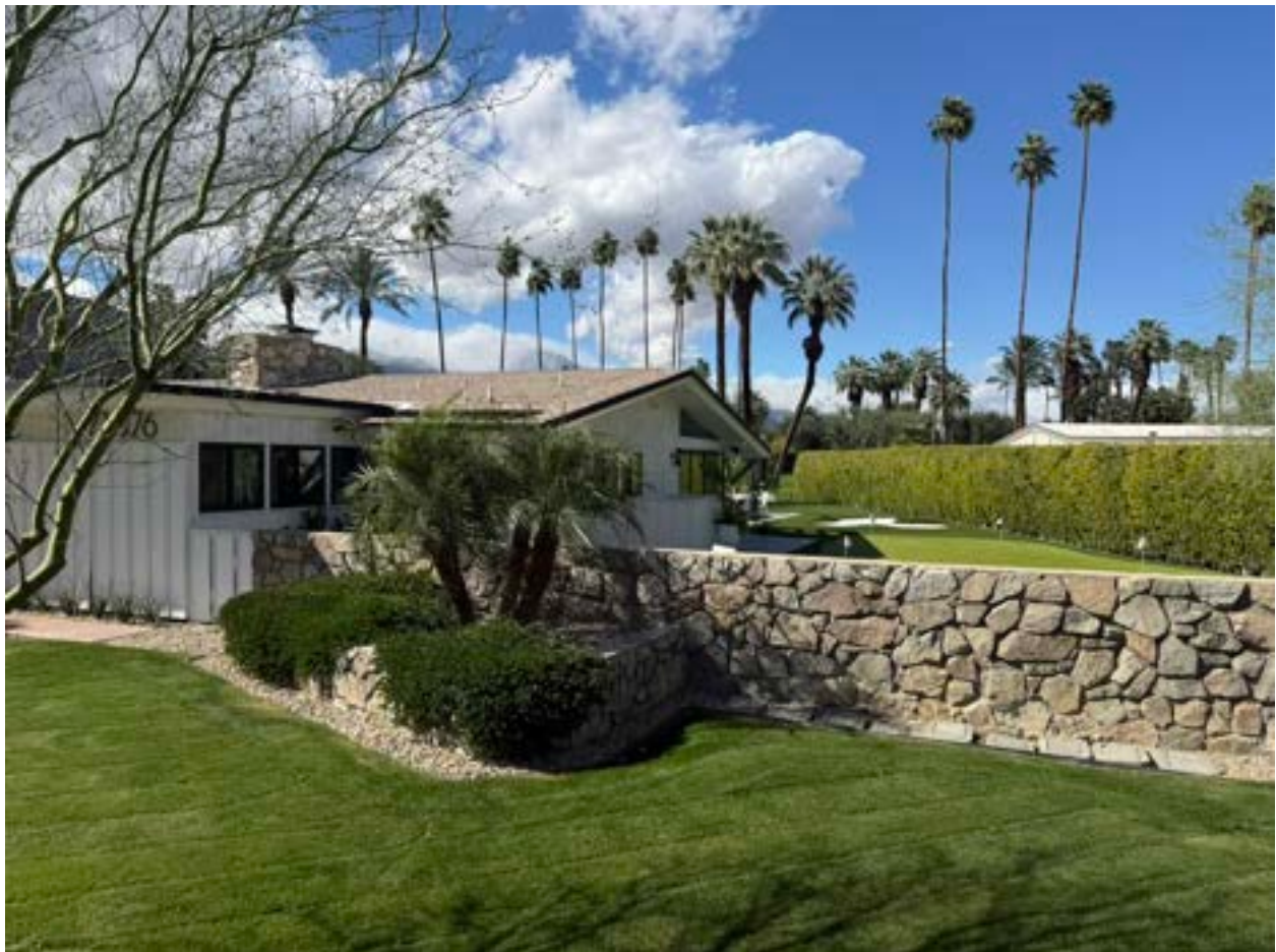
Board & batten siding detail, southeast corner, plus rock faced planters
