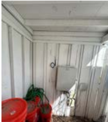
Northwest corner, equipment room with original board and batten siding
