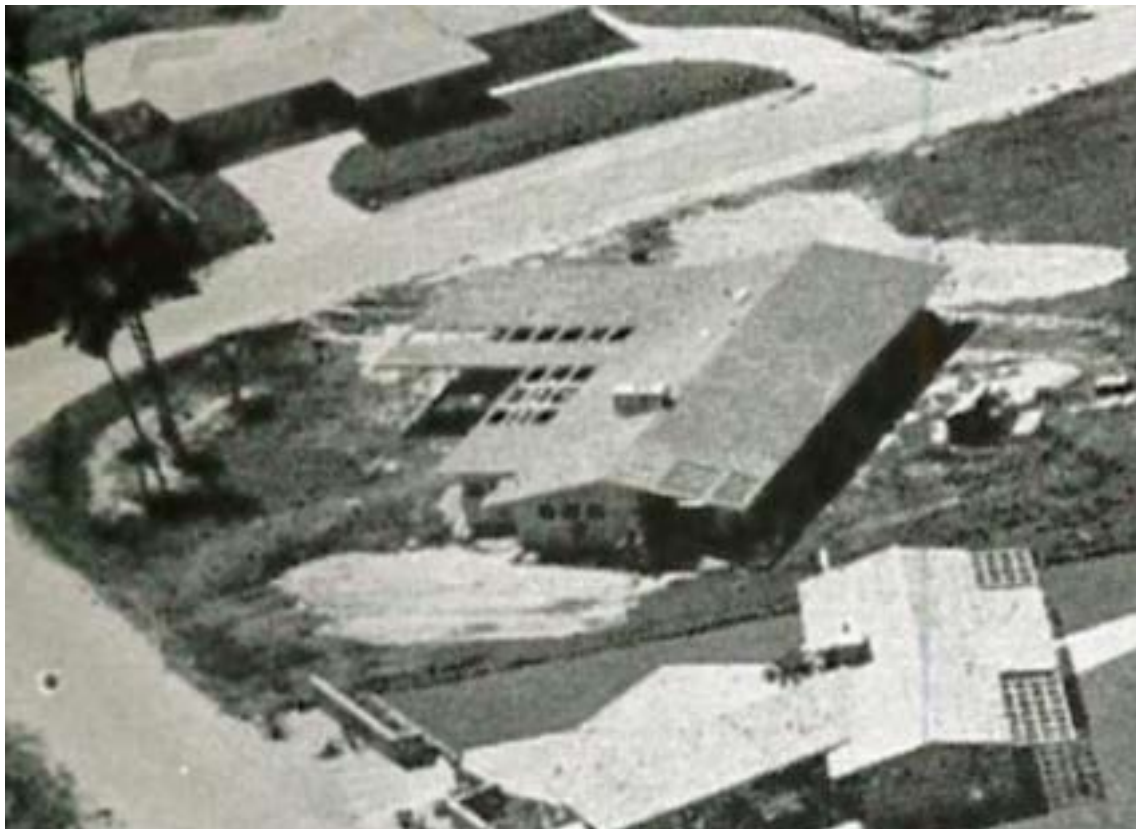
Close-up of image shown above, illustrates roof cut-outs in car port and to right of entry way
