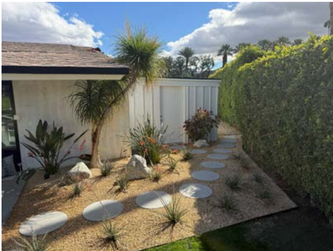
Northwest corner, looking southeast, shows doors and board and batten siding
