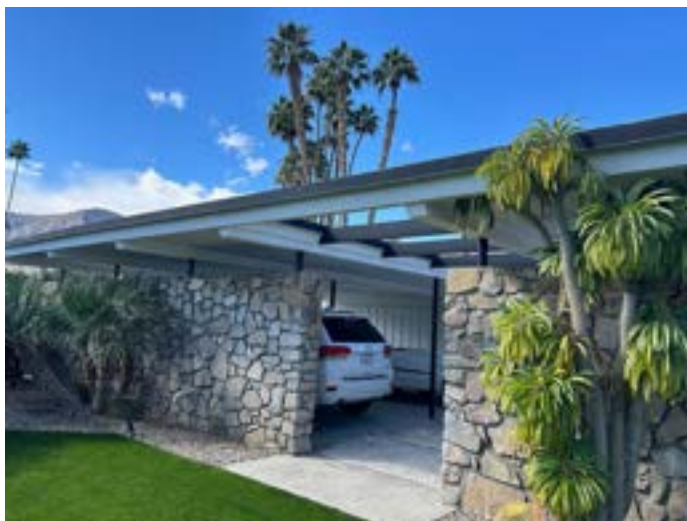
Porte cochere shows overhangs, lattice in roof, pathway, and opening between two rock-face walls, looking west
