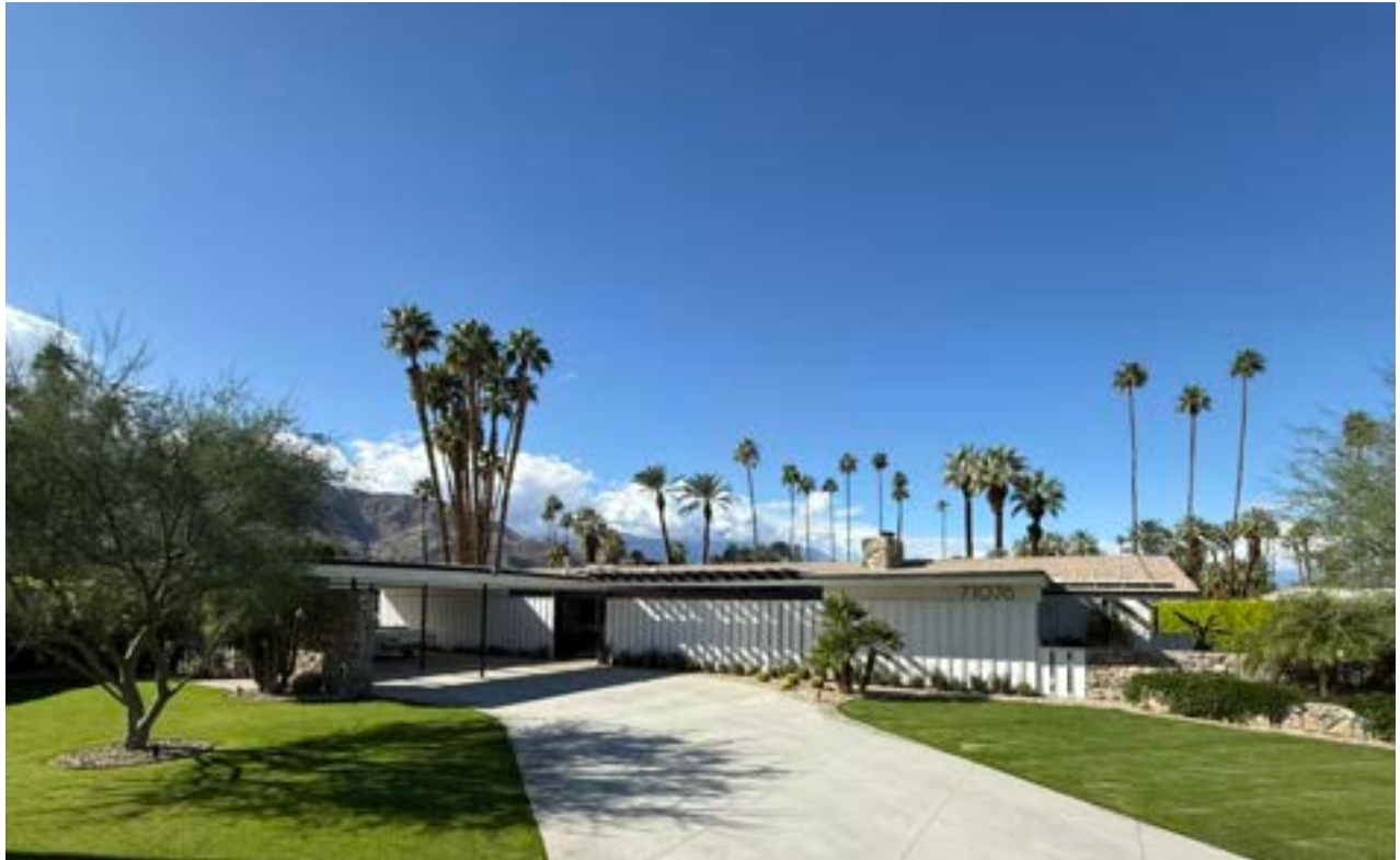
From Morning Springs Drive entry, looking west
