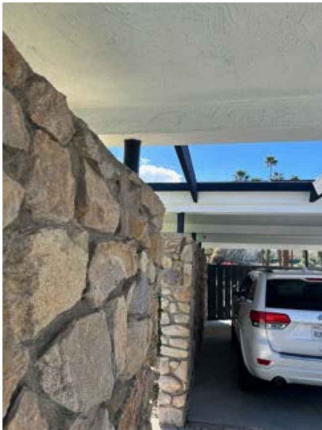
Porte cochere rock wall details and floating roof with lattice opening
