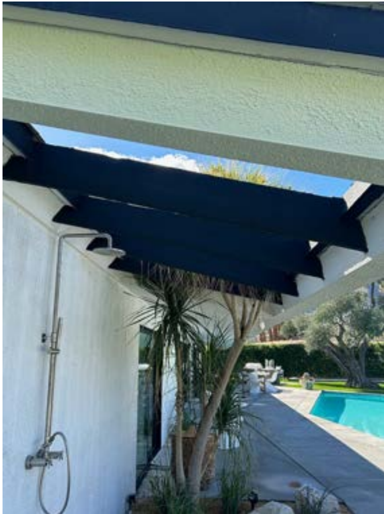
Northeast corner, roof opening as designed
