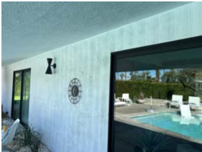
Vertically scored stucco appears on all elevations, here on the rear (north) elevation at the Simons Residence
