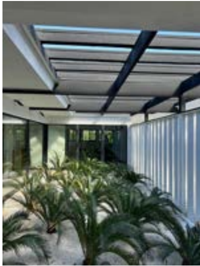
Lanai to right of entry shows overhang and latticed opening, vertical screen louvers
