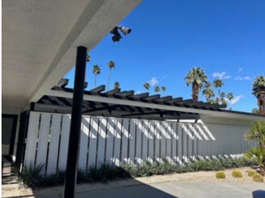
Covered walkway and narrow support; row of vertical louvers and lattice lanai to right of entry – looking northeast
