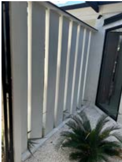
Vertical louvers to left of entry
