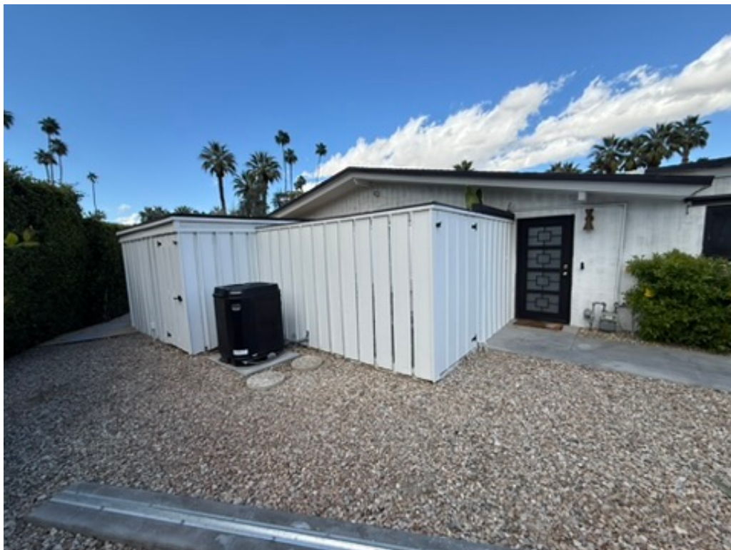
Vertical louvers repeat for equipment area
