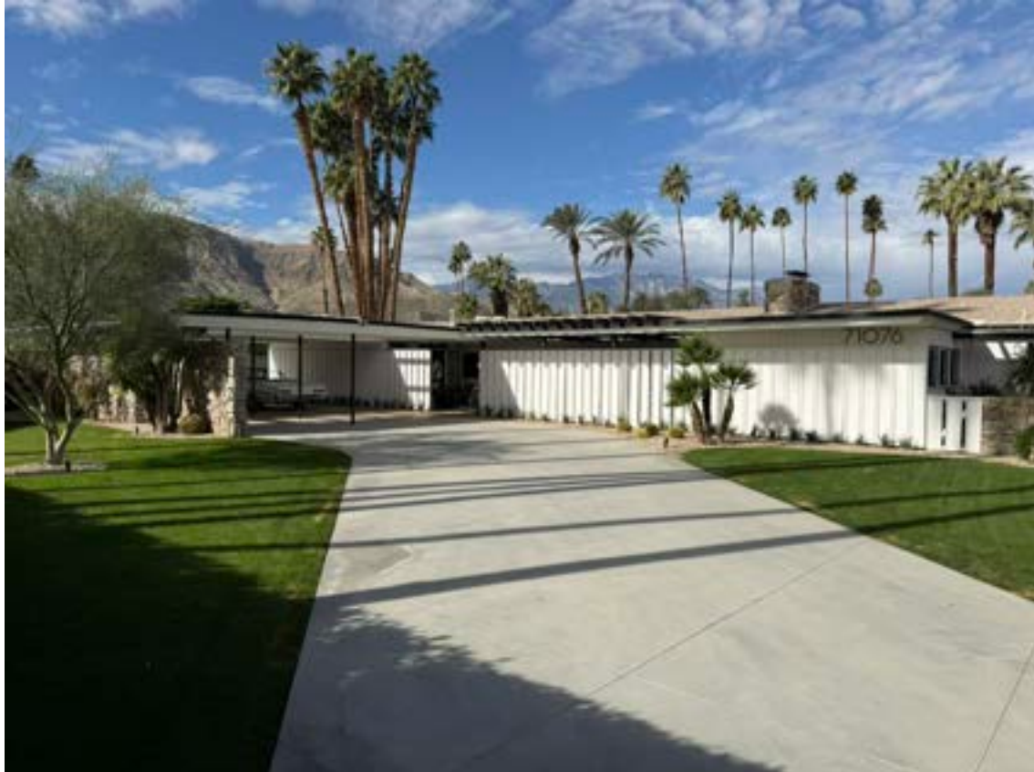
From Morning Springs Drive entry, looking west; east elevation shows two sets of triple windows and gable roofline
