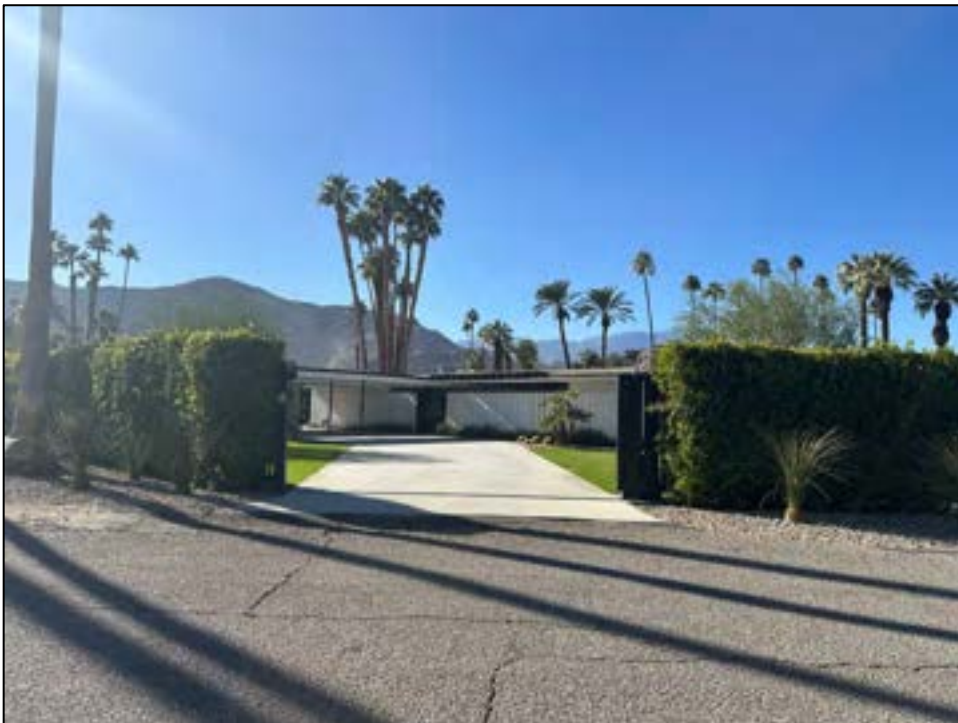
View of southeast (front) elevation. (71-076 Country Club Drive_1)
