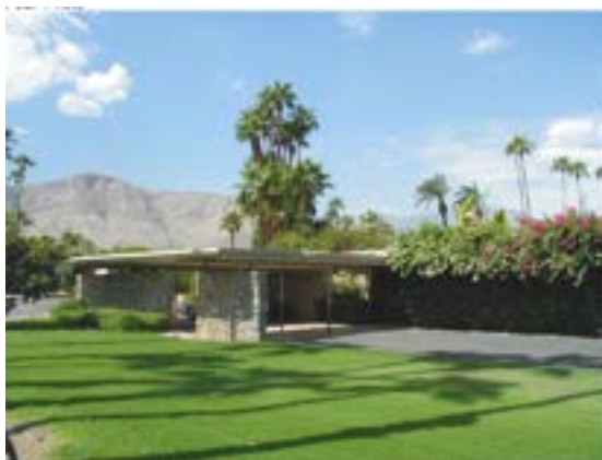
2002 photograph from DPR report
