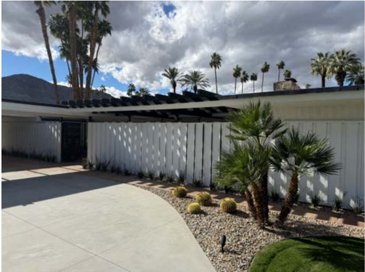
Porte cochere and row of louvers and board and batten siding to front elevation, looking west
