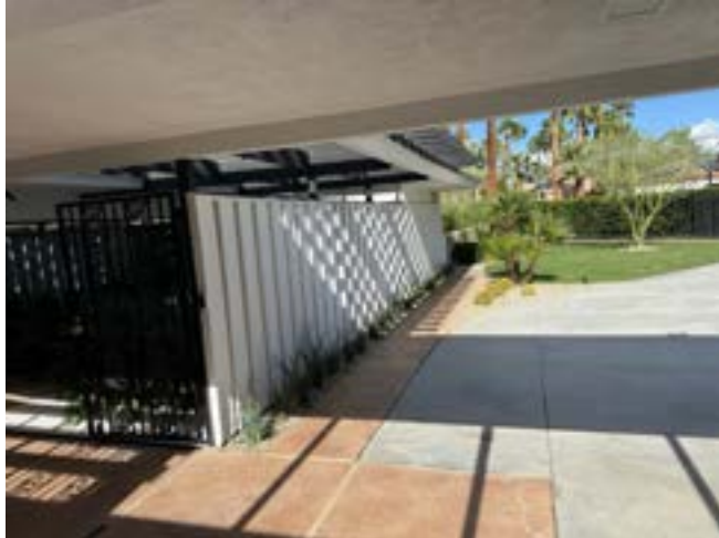
Vertical wood louvers screen the front lanai or sun court
