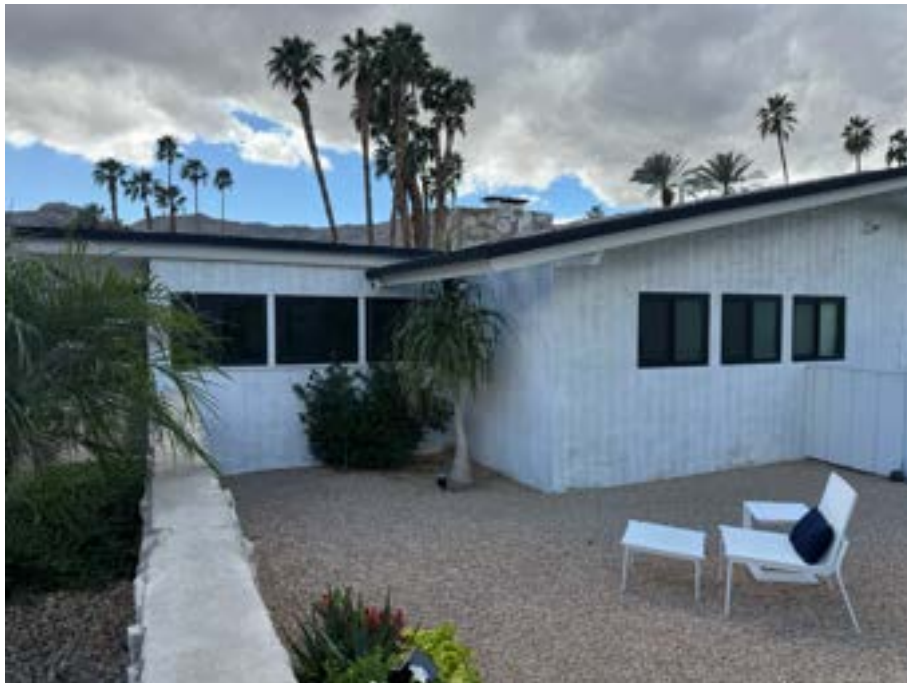
East elevation – looking west. Two rows of three windows as originally designed
