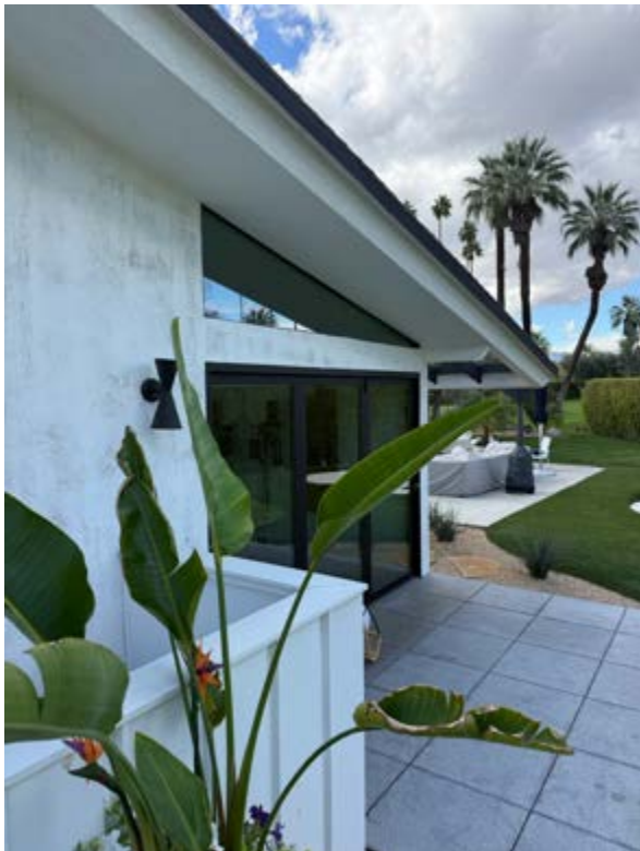
East elevation. Windows are not original
