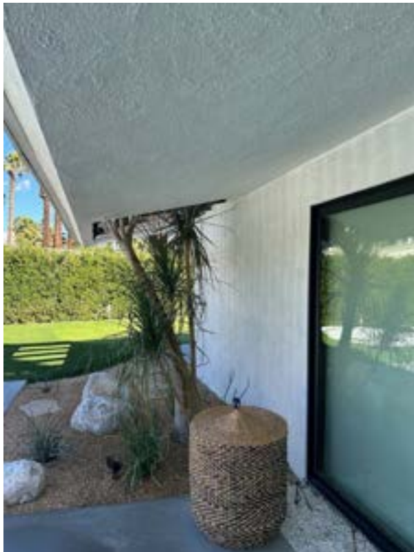
North east corner, looking east
