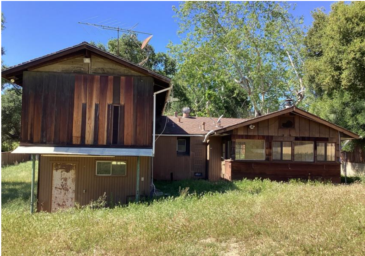
Rear/East Elevation (facing west)
