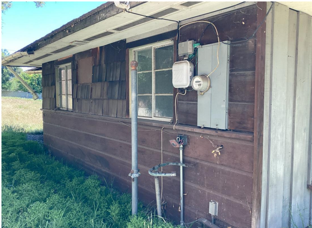
North Elevation (view of west section; facing southeast)
