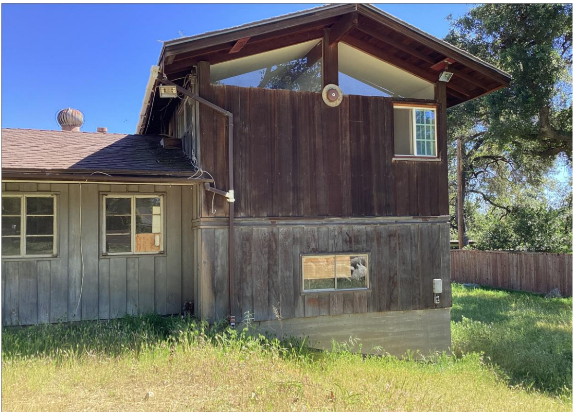
Primary/West Façade (view of south portion; facing east)
