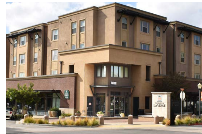
6.5: Building entry accentuated with corner location, wall articulation, projecting element and increased transparency
