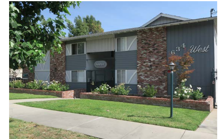
Older Garden Apartment Development in Sierra Madre
