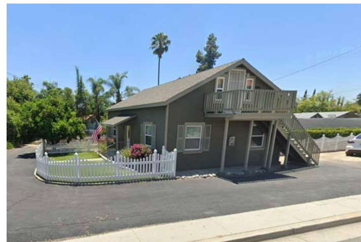
Lack of landscaping between the duplex and the street frontage.
