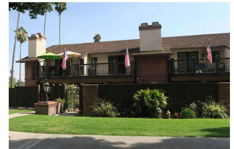
Survey of multifamily residential buildings in Sierra Madre
