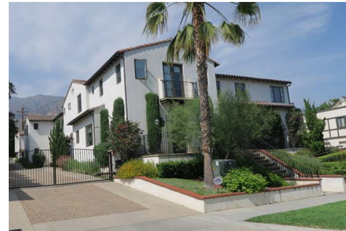
Survey of multifamily residential buildings in Sierra Madre
