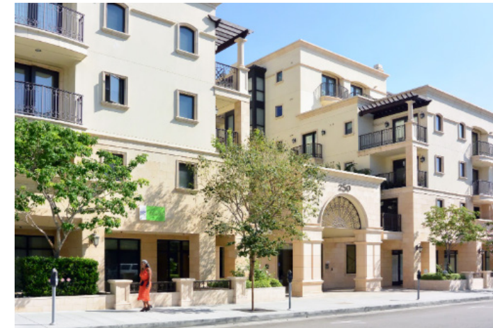
6.5: Building entry accentuated with wall articulation, massing break and portal interior courtyard
