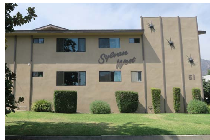
Lack of relationship between units and frontage
