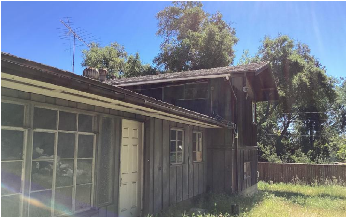
North Elevation (view of west portion; facing south)
