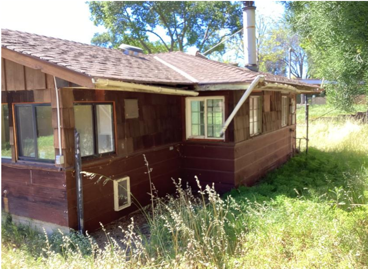
North Elevation (view of east section; facing west)
