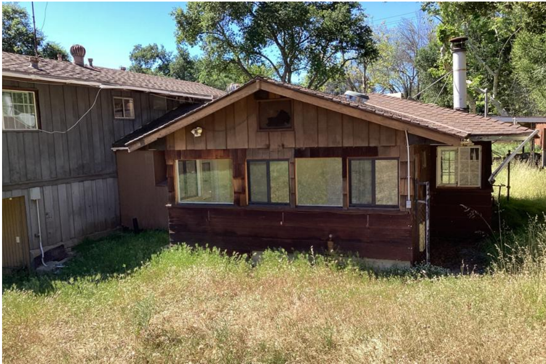
Rear/East Elevation (view of north sections; facing east)
