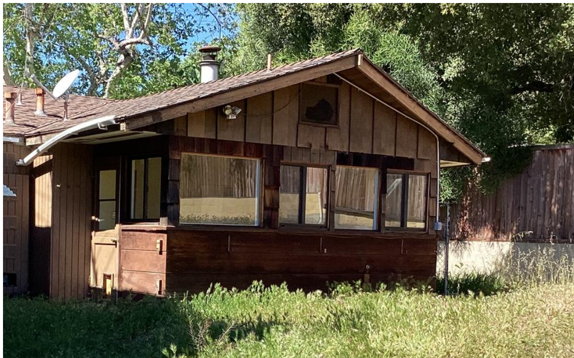
Rear/East Elevation (view of north portion; facing northwest)
