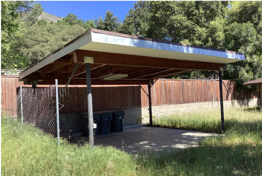
Carport (facing northeast)
