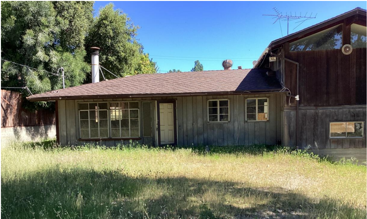
Primary/West Façade (view of north portion; facing east)
