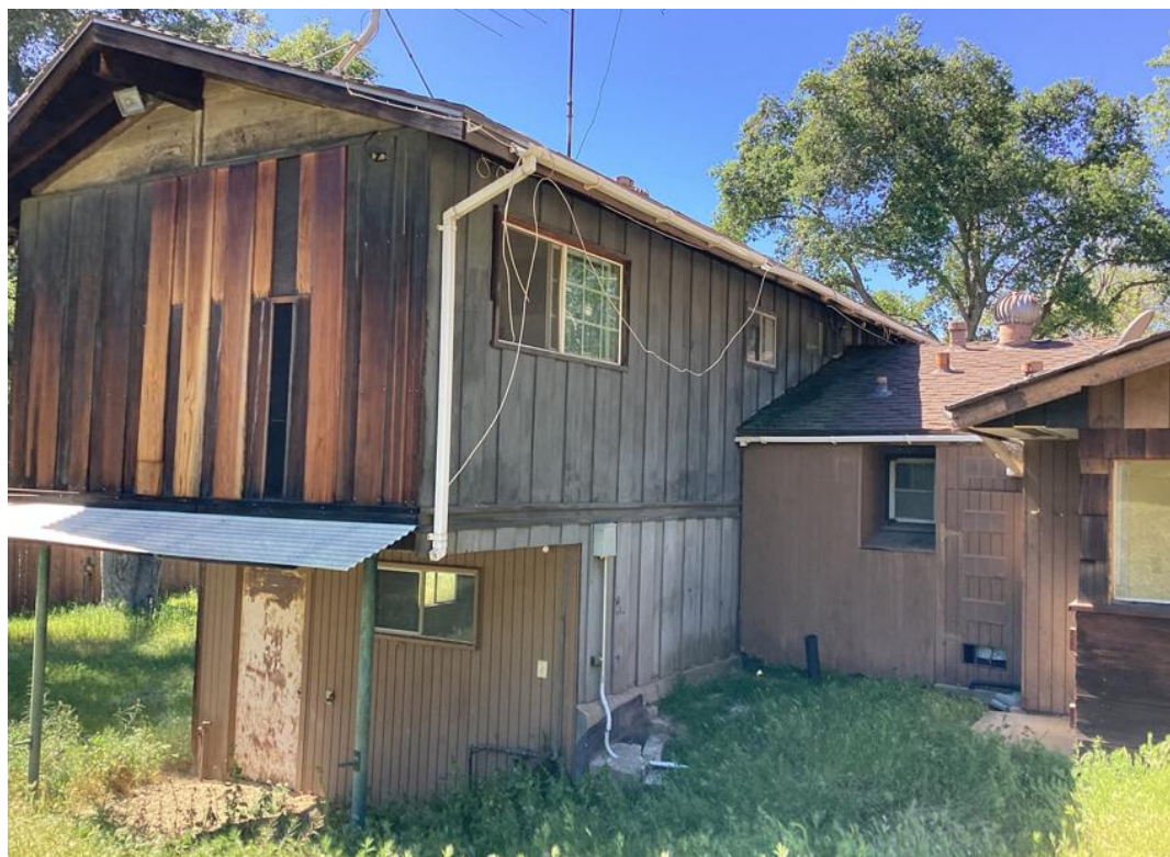
North Elevation (view of west portion; facing southeast)
